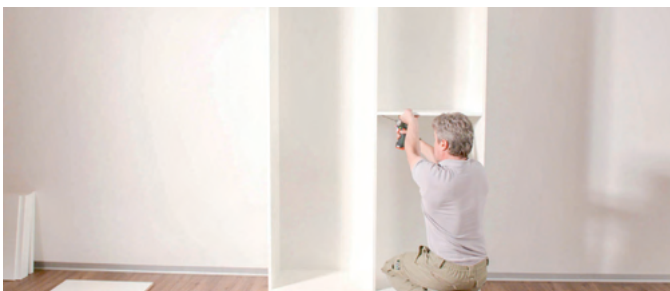
Screw front corner in place with a cordless drill. This makes one-man assembly easy.
