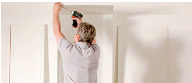
Screw front corner in place with a cordless drill. This makes one-man assembly easy.
